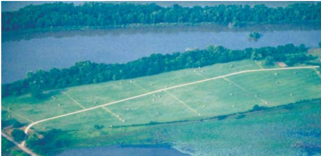
TCRWSS produces water for the system's six wholesale customers by pumping raw water from Lake Livingston through eighteen shallow wells located in natural sand and gravel deposits at the upper end of the lake. The well field, seen here, normally produces 1,100 gallons per minute. Production has been sharply reduced due to reduced water levels in Lake Livingston.
