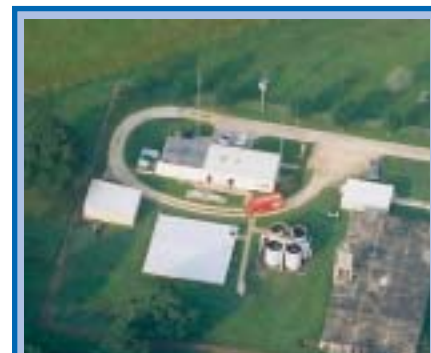
On the cover: The Trinity County Regional Water Supply System treatment plant. The Trinity River Authority has warned the wholesale customers of TCRWSS of an impending Water Shortage and Potential Loss of Supply as water production decreases and demands for water increase. The system's customers are urged to conserve water and be prepared to implement their drought contingency plans. See Story, this page.
